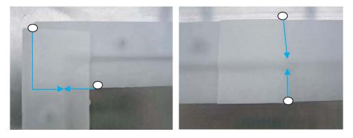
In the above images, the white circles indicate where 3M 4000UV should be applied in the corner and step situations. These two general categories can describe most common configurations. For configurations other than these, the general principle is to use  $3M^{TM}$  4000UV in any place where water (shown as blue arrows) could seep past an improperly joined overlap.
